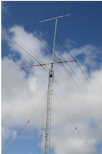
The 4 element 50MHz LFA-LN installed at ZD7VC
