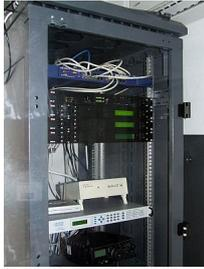
Controller unit to allow the control of many rotator devices via Ethernet connection
