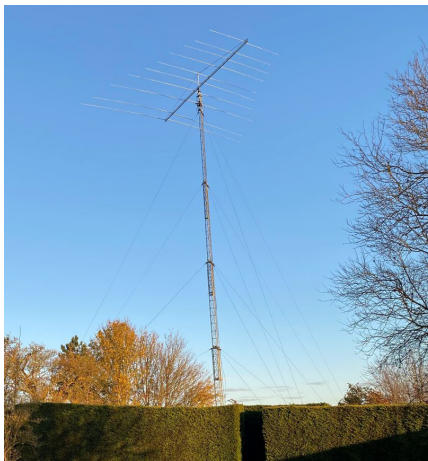
The BOLPA at G2YT - installed at 85'
