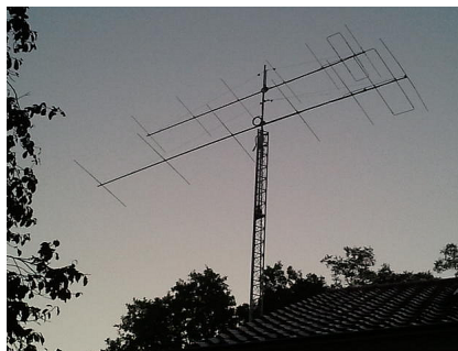
A 7el 70MHz LFA installed above a 7el 50MHz LFA at PA7F
