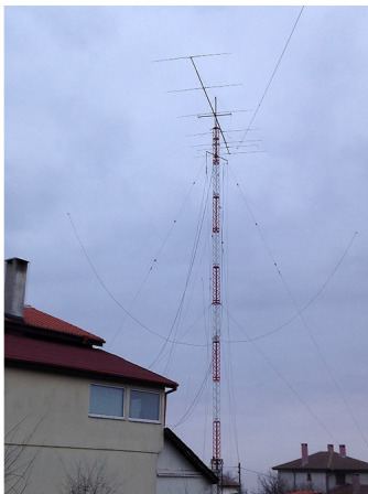
The 7 element OP-DES for 28MHz at LZ4TX
