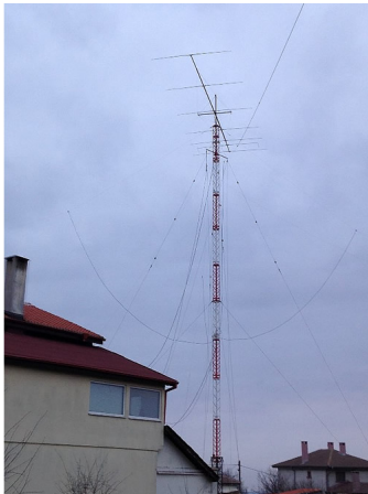
The 7 element OP-DES for 28MHz at LZ4TX
