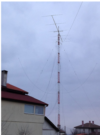
The 7 element OP-DES for 27/28MHz at LZ4TX
