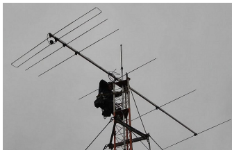
The 6R6 6 element 50MHz LFA-R being installed by XE2K
