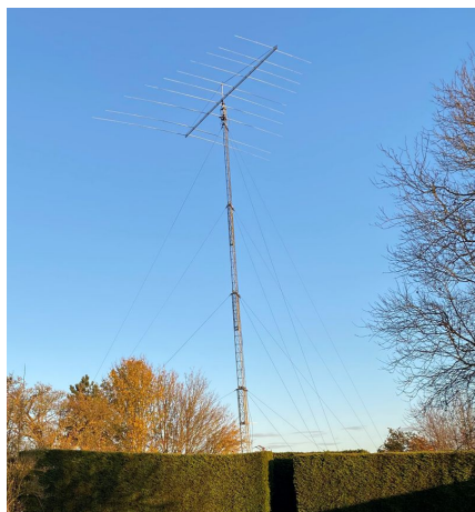
The BOLPA at G2YT - installed at 85'
