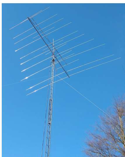
Installed at G1XOW
