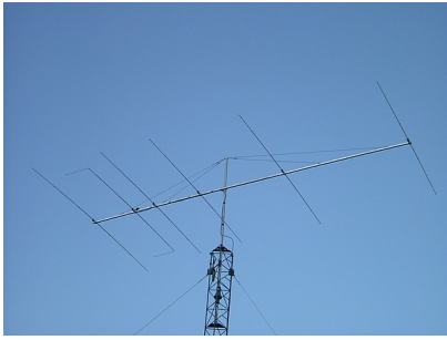
A 6el 27MHz OP-DES installed in Norway
