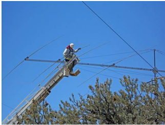
A 6el 20m OP-DES being installed at K5RC
