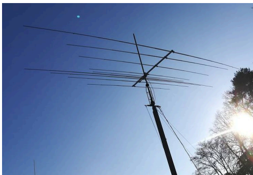
The XR5 installed at club station G8VGG
