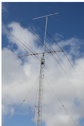
The 4 element 50MHz LFA-LN installed at ZD7VC
