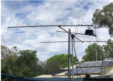
A pair installed at VK6JX
