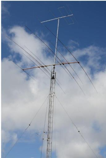
The 4 element 50MHz LFA-LN installed at ZD7VC
