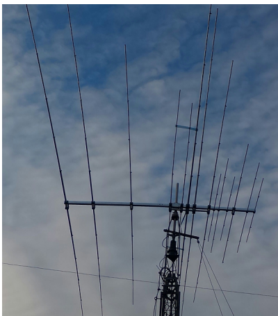
The XR7 installed at G0MTQ
