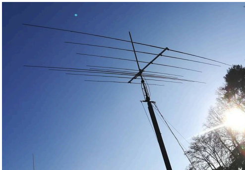
The XR5 installed at club station G8VGG
