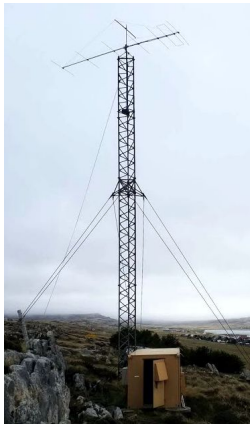
A single 7el 50MHz WOS in use at VP8EME reflecting signals off of the Moon
