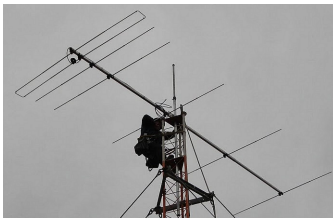
The 6R6 6 element 50MHz LFA-R being installed by XE2K
