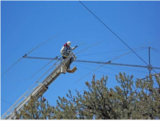
A 6el 20m OP-DES being installed at K5RC
