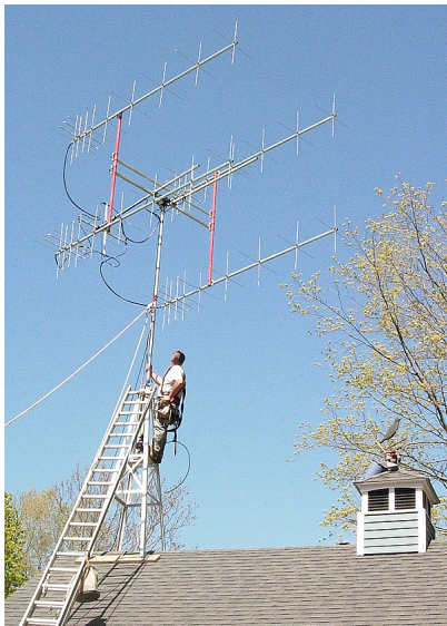
4 x 8V/8H X-pol LFAs on InnovAntennas fully insulated (vertical sections) H-frame
