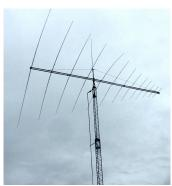
The 10-54MHz LDPA directional antenna at K4ANP. Sadly, Len caught one of the elements and bent it during installation but SWR 1:1.4 thorughout.
