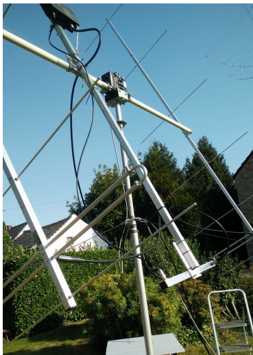
A pair of 7el OWL Ultra's being installed at ON4EC
