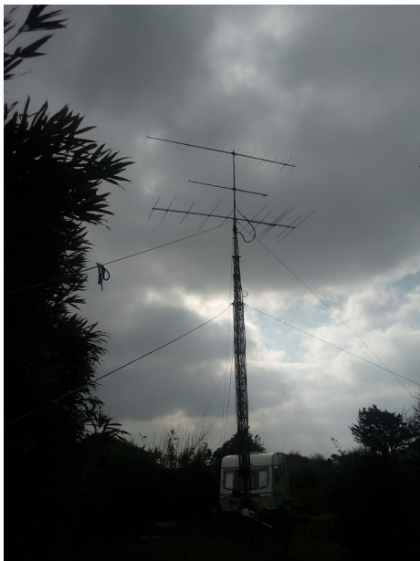
Above - the 12el installed at G7RAU
