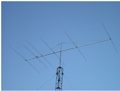
A 6el 27MHz OP-DES installed in Norway
