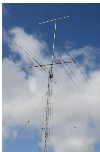
The 4 element 50MHz LFA-LN installed at ZD7VC
