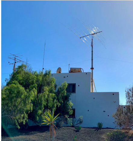
The XR7 installed at EA8BFK
