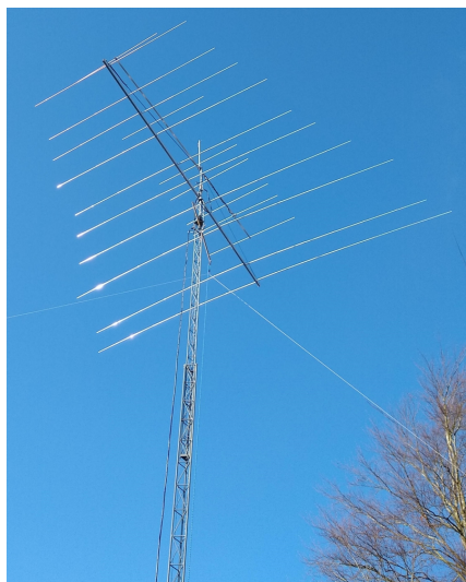
Installed at G1XOW
