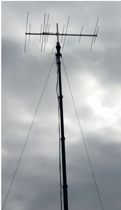
The 12el Duo installed at M0VOZ
